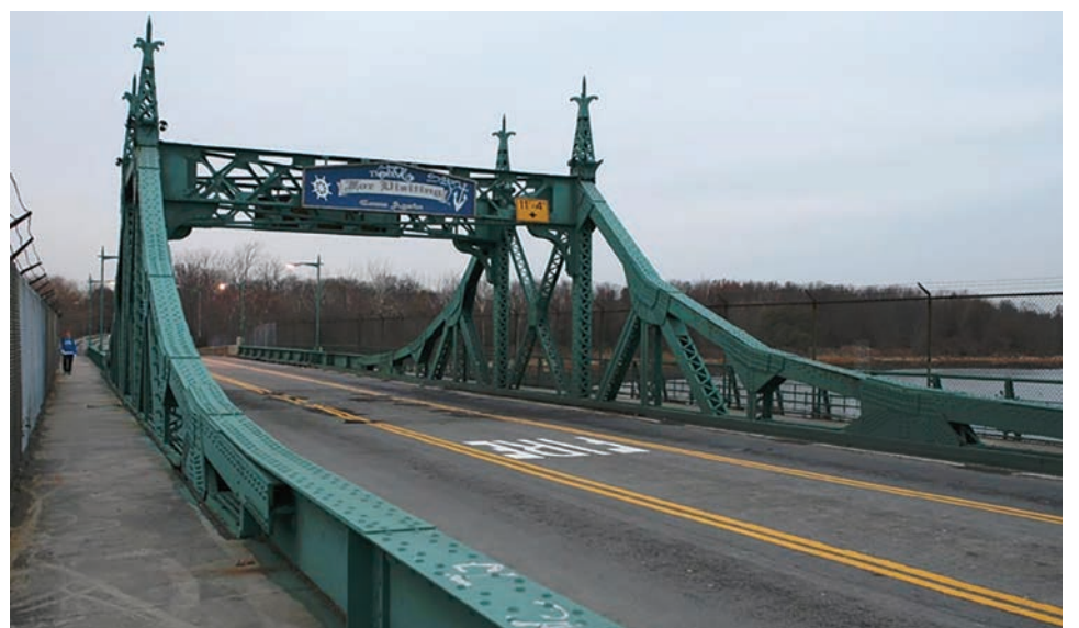
The second City Island bridge, built in 1901, was slated for demolition in 1999.
