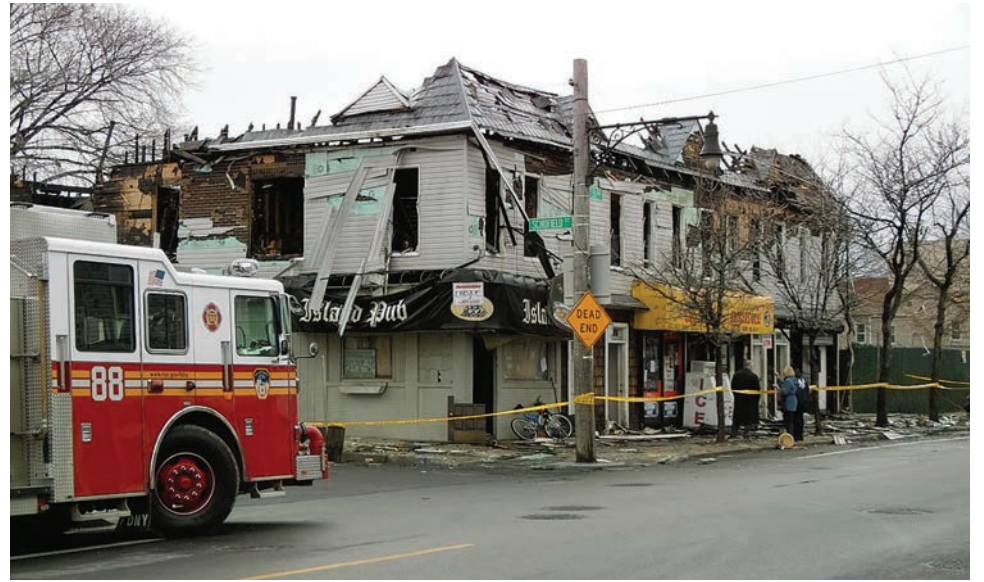
The row of buildings featuring the Island Pub on City Island Avenue at Schofield Street burned in 2006.
