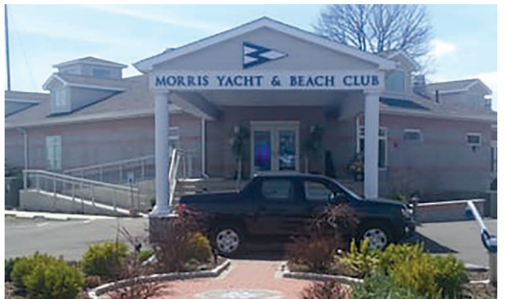
In June 2009, the Morris Yacht Club broke ground for this new, modern building.
