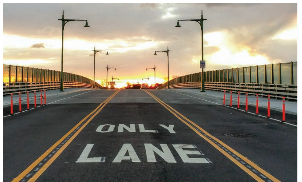
The new bridge was in the process of construction for several years but finally opened in 2017.
